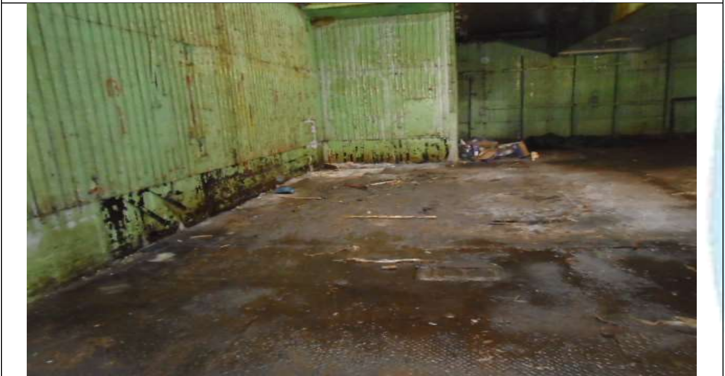
CARGO HOLD BULKHEAD
